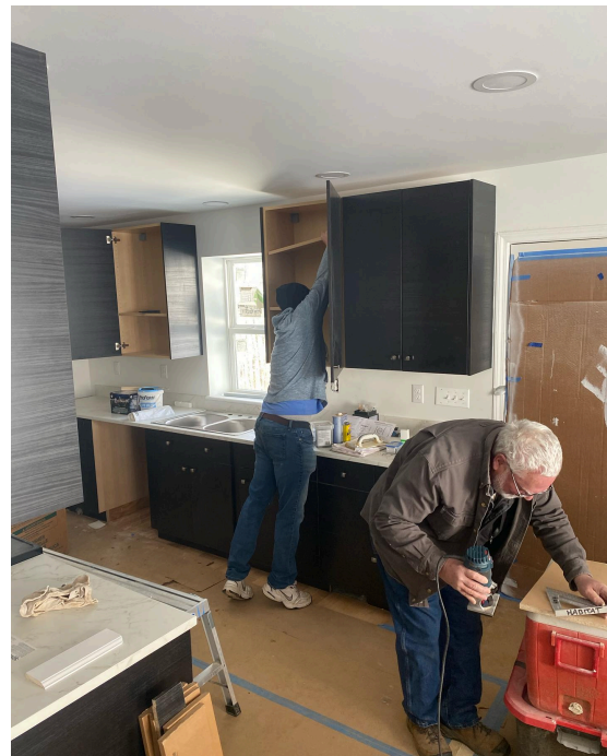
These gorgeous kitchen cabinets are now fully installed!
