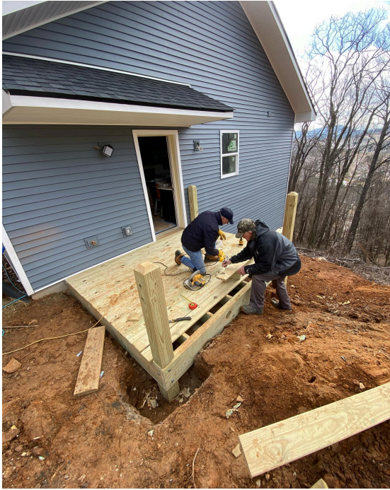
Working on a safe entry for our partner family
