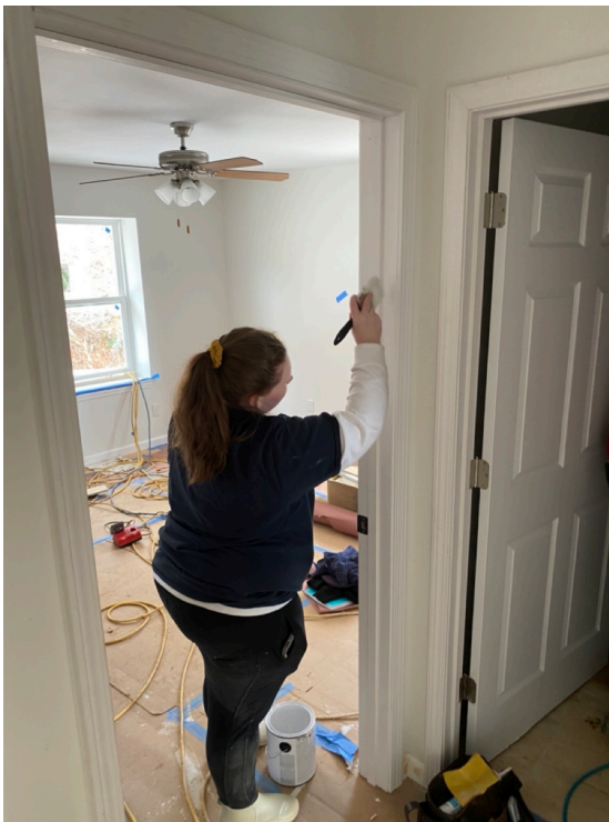
Interior trim is painted!
