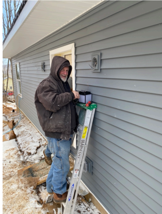
Exterior lighting installation
