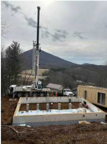
Crane in place and ready to lift the house
