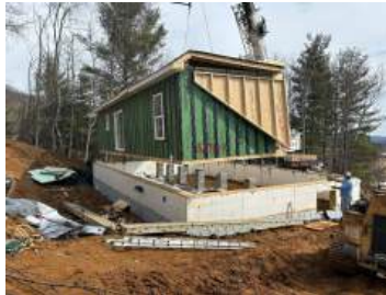
First section almost in place
