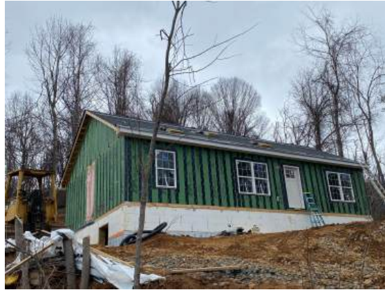
Our first modular home in place and ready to finish!
