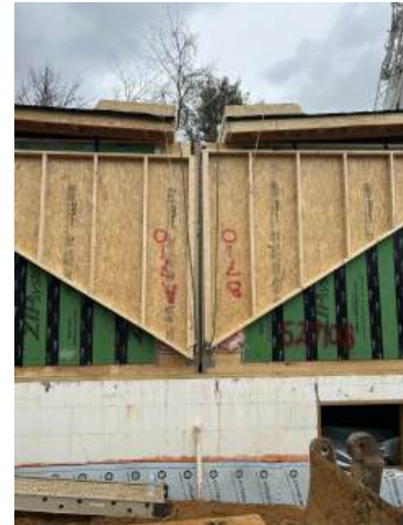
Both sections in place and ready to be joined
